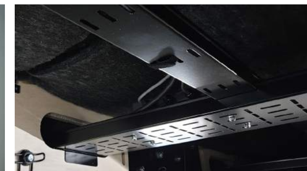
Cable-management within ceiling
